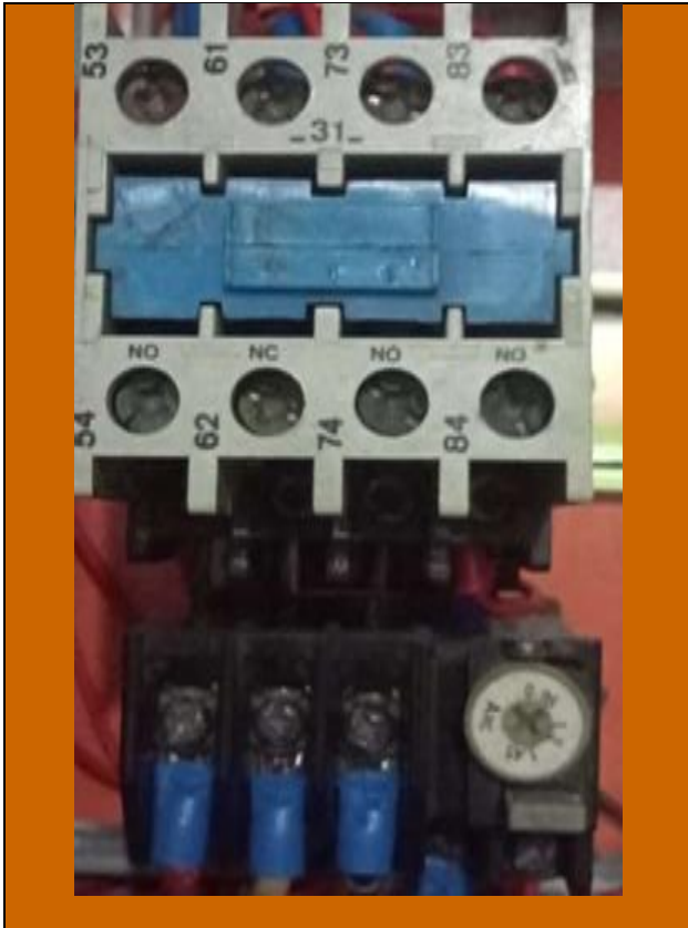
Figure 10: Magnetic Contactor and Over Load
